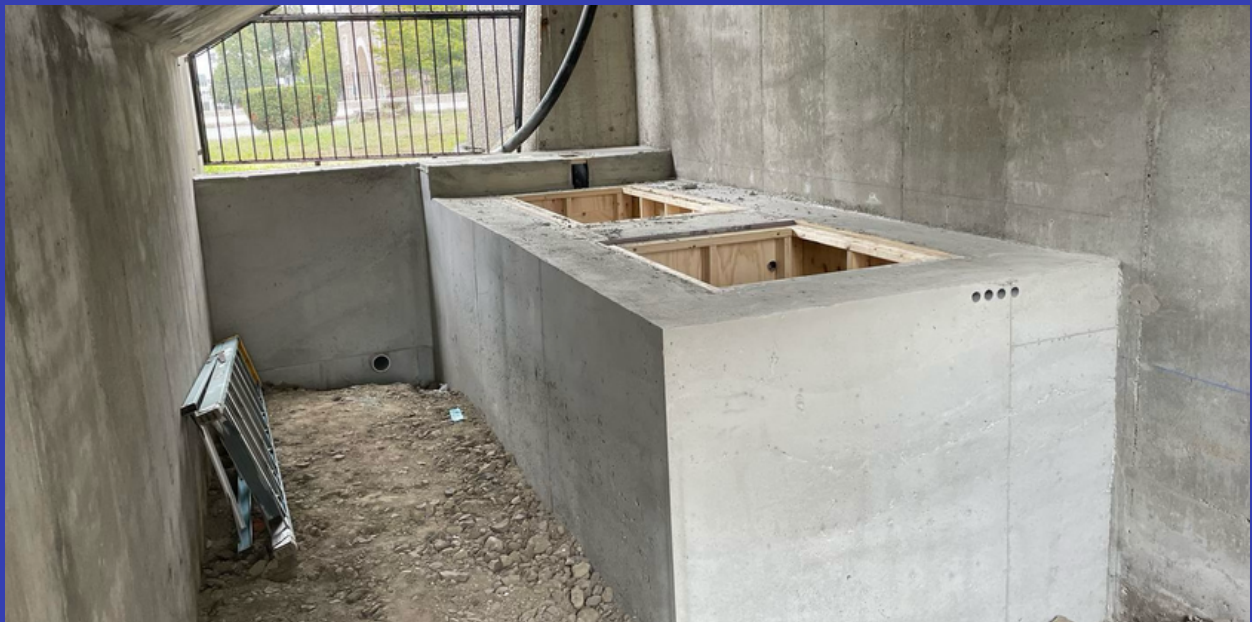
The concrete for a new dish mikvah, poured this year by Matrix Concrete — the same contractor that built our original mikvah.
